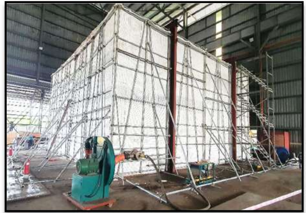
PWHT FURNACE (GAS FIRING) TPG JETTY 12mW x 12mL x 6mH
