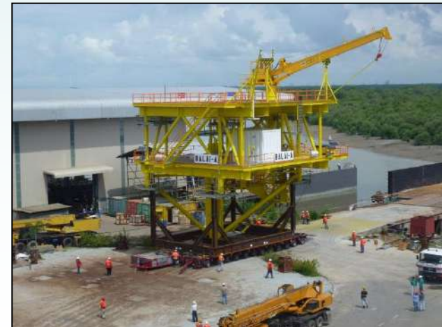
Balai platform load out
