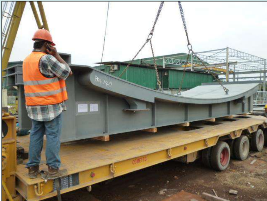
Delivery Bottom Plate Saddle to Port Klang
