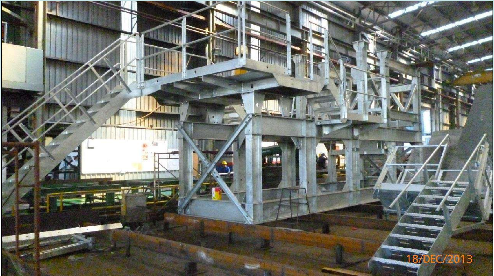
MJ 42A Base Structure
