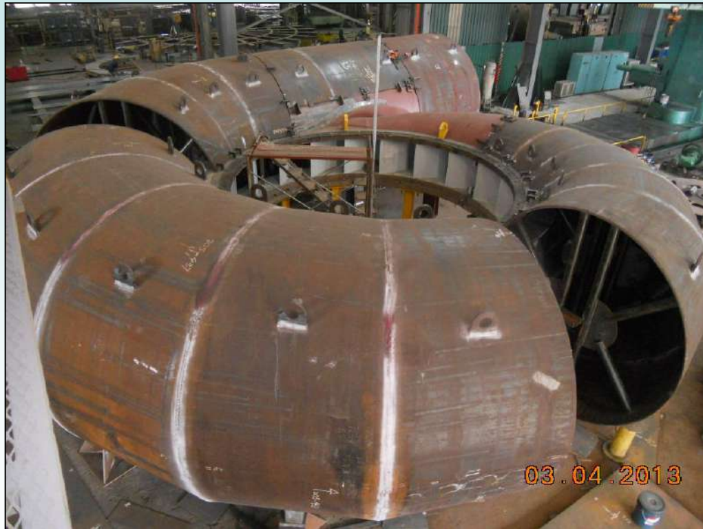
Spiral Case and Embedded Parts - Completed July 2013
