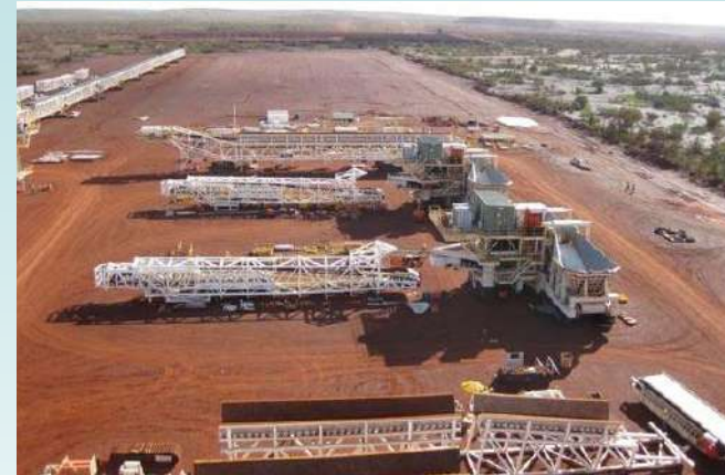
Bridge 45 & System #1 TTMSs
