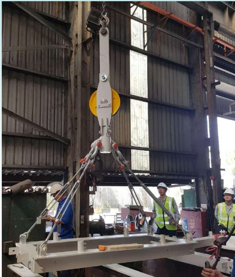
Temporary Hanging Scaffolding Setting
