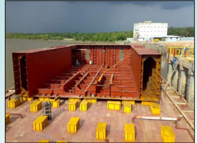
Hull Assemble on Floating Dock
