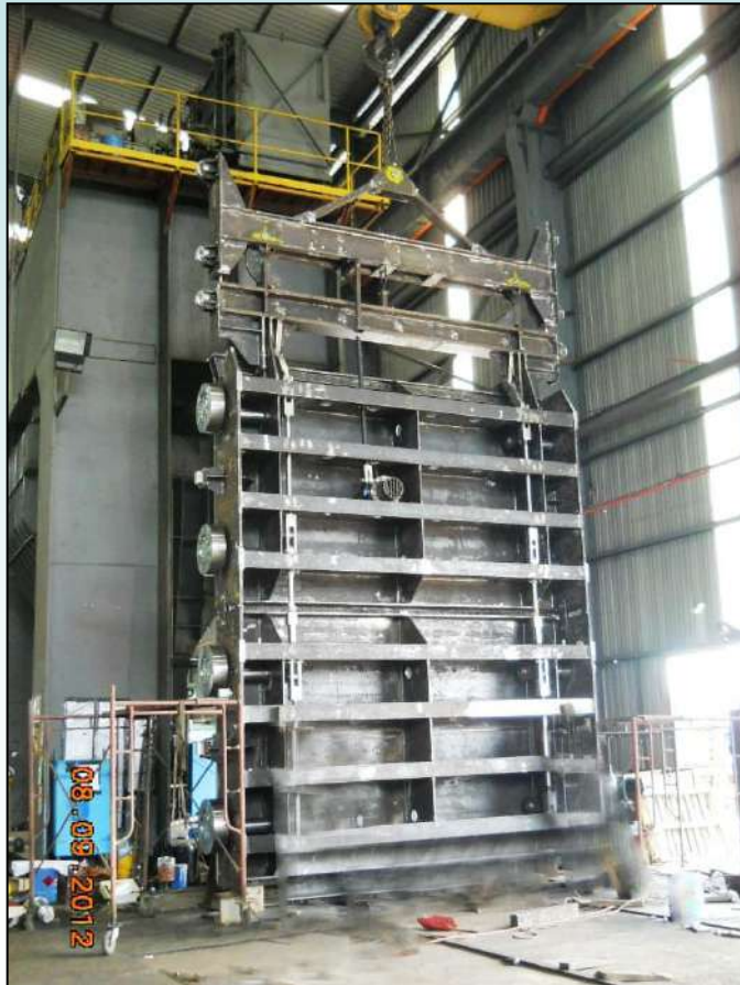
Diversion Tunnel Stoplogs -Completed Oct 2012
