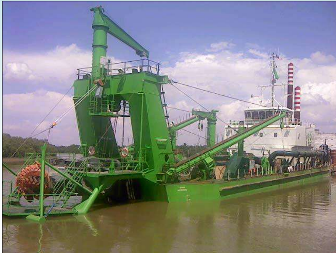
Construction of GANGA CSD 750S (Mono Hull)
