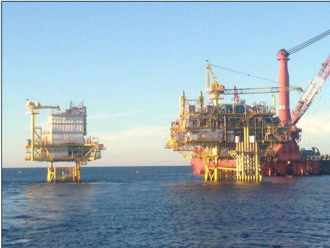
Living Quarter installed at site
