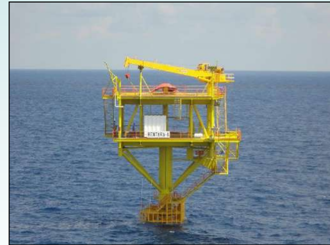
Bentara Topside site installation
